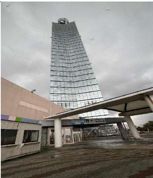
Photo 17 Port Tower "Serion"
